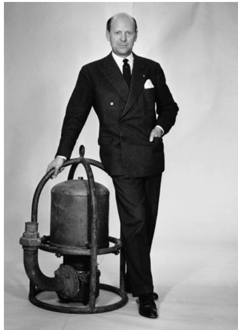
Figure 2. The worlds first submersible drainage pump, accompanied by its inventor Sixten Englesson.
